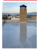
One component liquid waterproofing composition, after polymerization gives an elastomeric, cold-applied polyurethane membrane.
